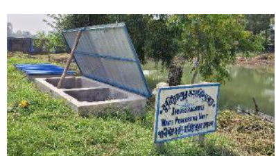
Waste Processing Unit
